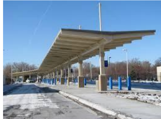
North Omaha Transit Canopy Structure
