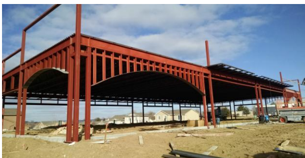
Retail Structure with Lintel Beam and Plate
